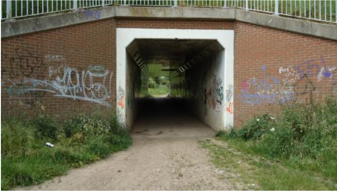
Tunnel under The Dove Way at the western edge of the site
