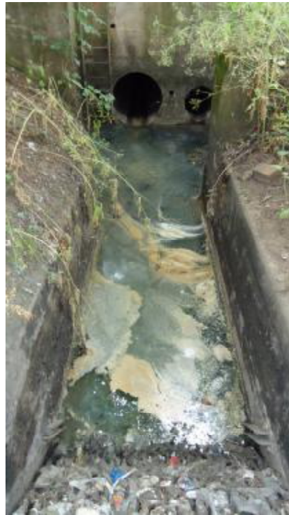
The Wharf Brook at the discharge point and end of the culvert in the western section of the site
