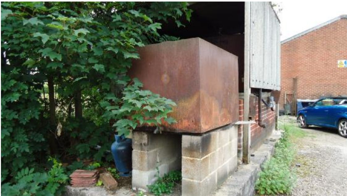
ASTs adjacent to the vehicle repair works
